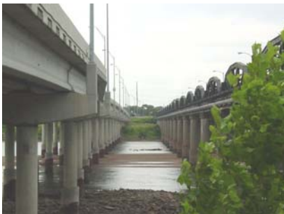
View between 96 th Street Bridge and Pedestrian Bridge at Jenks
