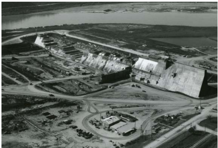
1961 Photograph of Keystone Dam under construction
