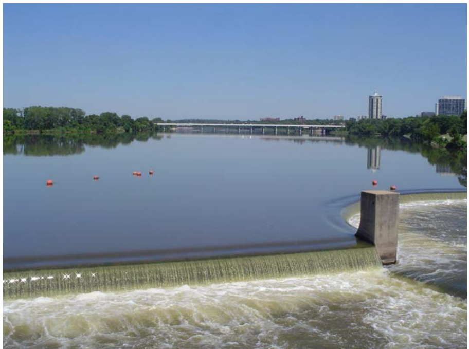
Water flowing over the ogee weir at Zink Lake
