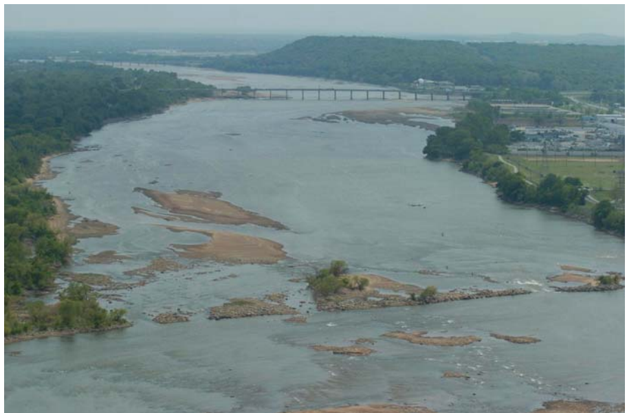
Looking south along the Arkansas River toward Turkey Mountain
